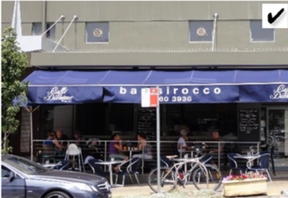
Canvas materials are permitted as awning extensions and they should be fixed to the underside of the awning.
