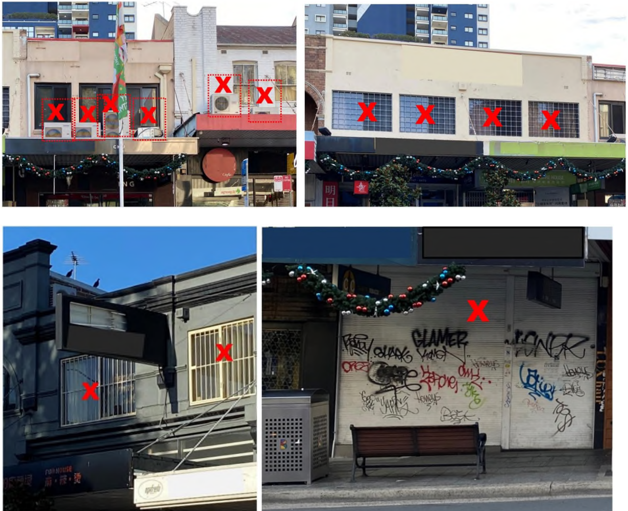
Figure 7. Examples of prohibited security bars, shutters or permanent grilles and air handling systems
