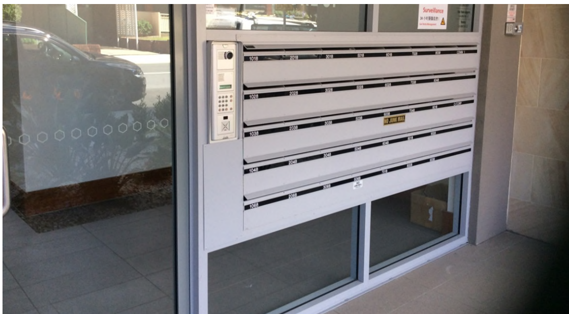
Figure 1. Examples of Mailboxes Integrated into the Front Wall of a Residential Flat Building
