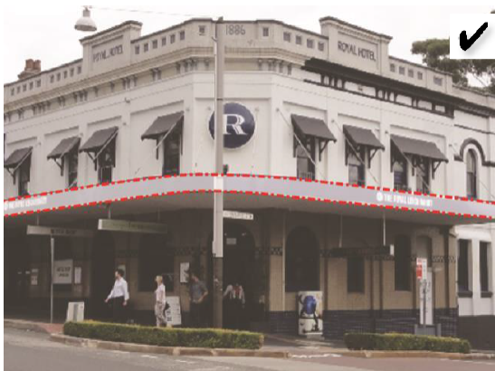
Continuous splayed awning around the corner
