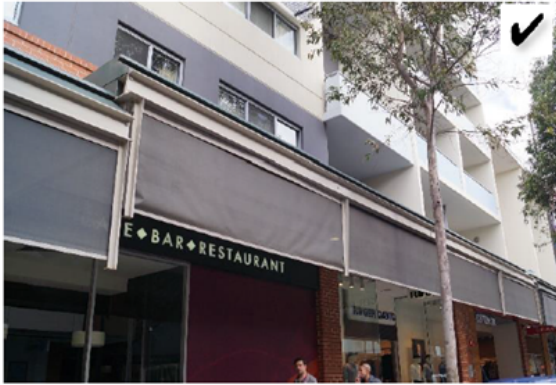
Retractable partial drop down awning extensions that are fixed to the underside of the fascia and in a coordinated colour scheme
