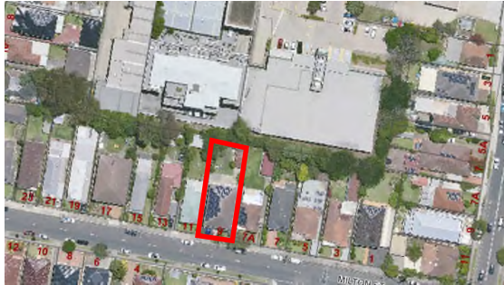
Figure 62 - Aerial image of the subject site Nos.9 Milton St (outlined in red)
