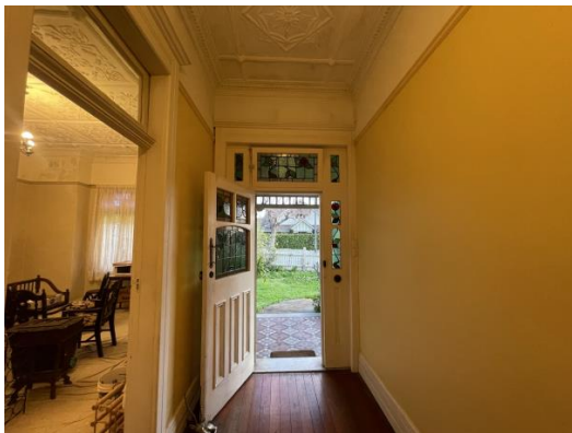
Figure 4.57 27 Woodside Avenue – front entry
