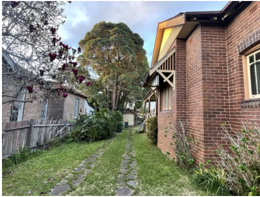
Figure 4.19 25 Woodside Avenue- western elevation
