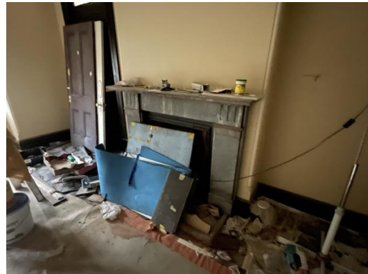
Figure 4.26 25 Woodside Avenue – marble fireplace
