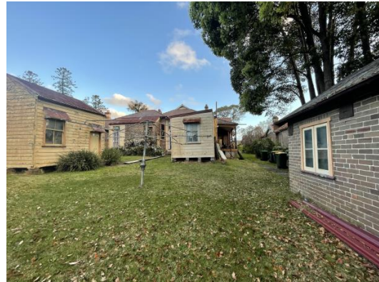
Figure 4.40 25 Woodside Avenue – rear of house
