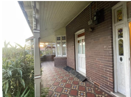
Figure 4.54 27 Woodside Avenue - verandah
