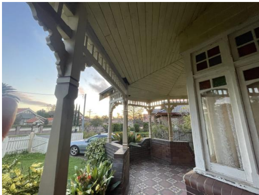
Figure 4.53 27 Woodside Avenue - verandah
