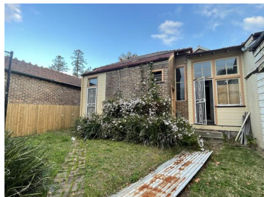
Figure 4.44 25 Woodside Avenue – rear of house
