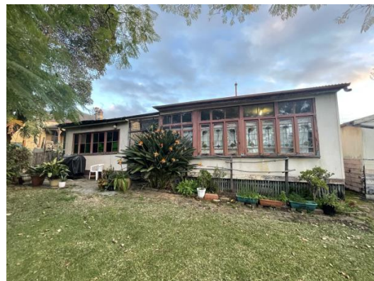
Figure 4.72 27 Woodside Avenue – rear of house
