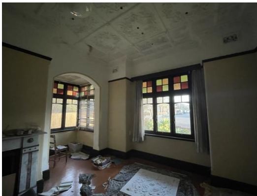
Figure 4.31 25 Woodside Avenue – front reception room
