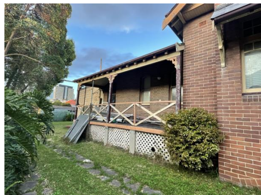
Figure 4.18 25 Woodside Avenue – western verandah
