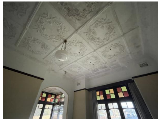
Figure 4.32 25 Woodside Avenue – ceiling detail
