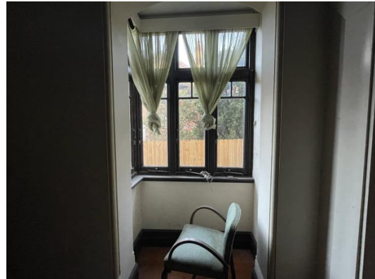
Figure 4.34 25 Woodside Avenue – window detail
