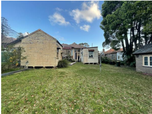
Figure 4.39 25 Woodside Avenue – rear of house
