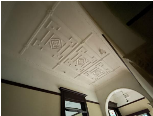
Figure 4.27 25 Woodside Avenue – ceiling detail
