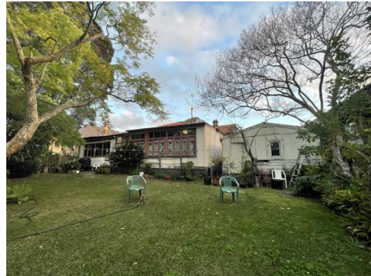
Figure 4.74 27 Woodside Avenue – rear of house and garage
