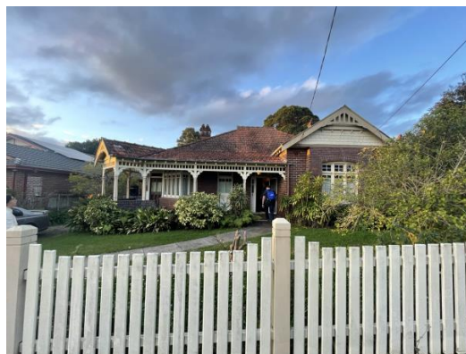
Figure 4.48 27 Woodside Avenue – front facade
