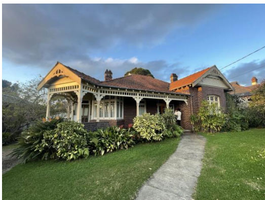
Figure 4.47 27 Woodside Avenue – front facade
