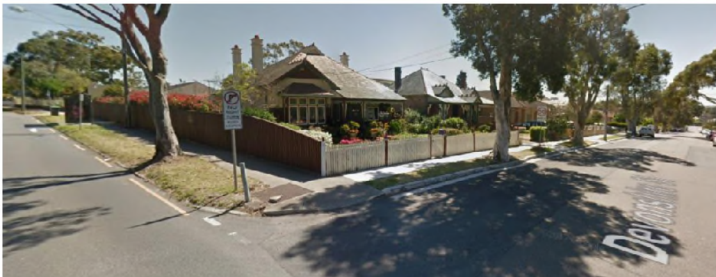
Property at 35 Devonshire Street Croydon
