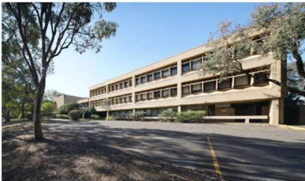
Picture 9 – Existing Building Photograph
