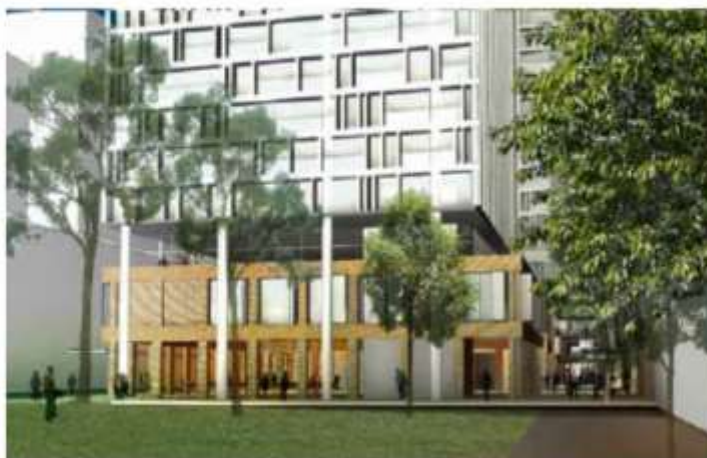
Figure 3-10 View of current building form from the Council car park
