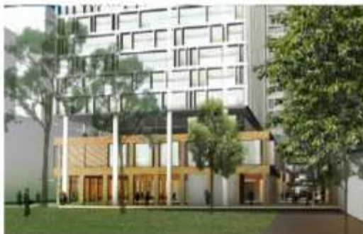
Figure 3-13 Current PP Building D viewed from Council car park in Railway Pde
