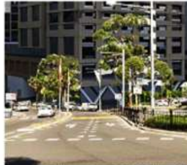
Figure 3-14 April 2018 Amended PP Building D viewed from Roundabout in Railway Pde
