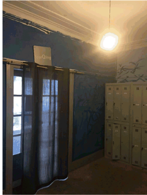
Picture 8 – View of an internal room on the first-floor Source: Urbis
