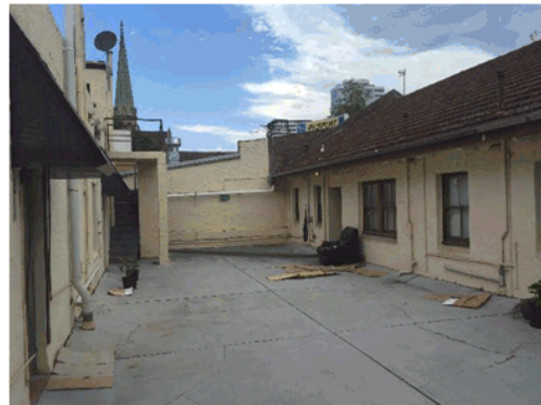
Picture 4 – View of the first-floor terrace Source: Urbis
