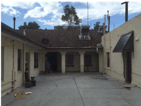
Picture 5 – View of the first-floor terrace Source: Urbis
