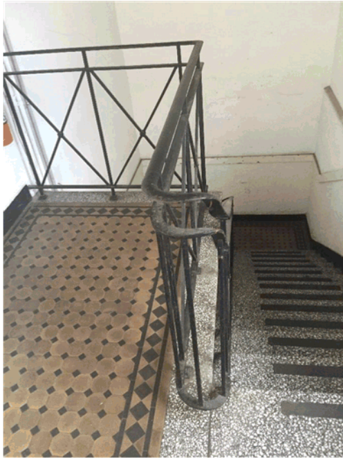
Picture 7 – View of the internal staircase Source: Urbis
