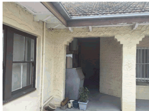
Picture 6 – View of the first-floor terrace Source: Urbis
