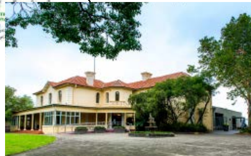
Woodstock Community Centre Upgrade
